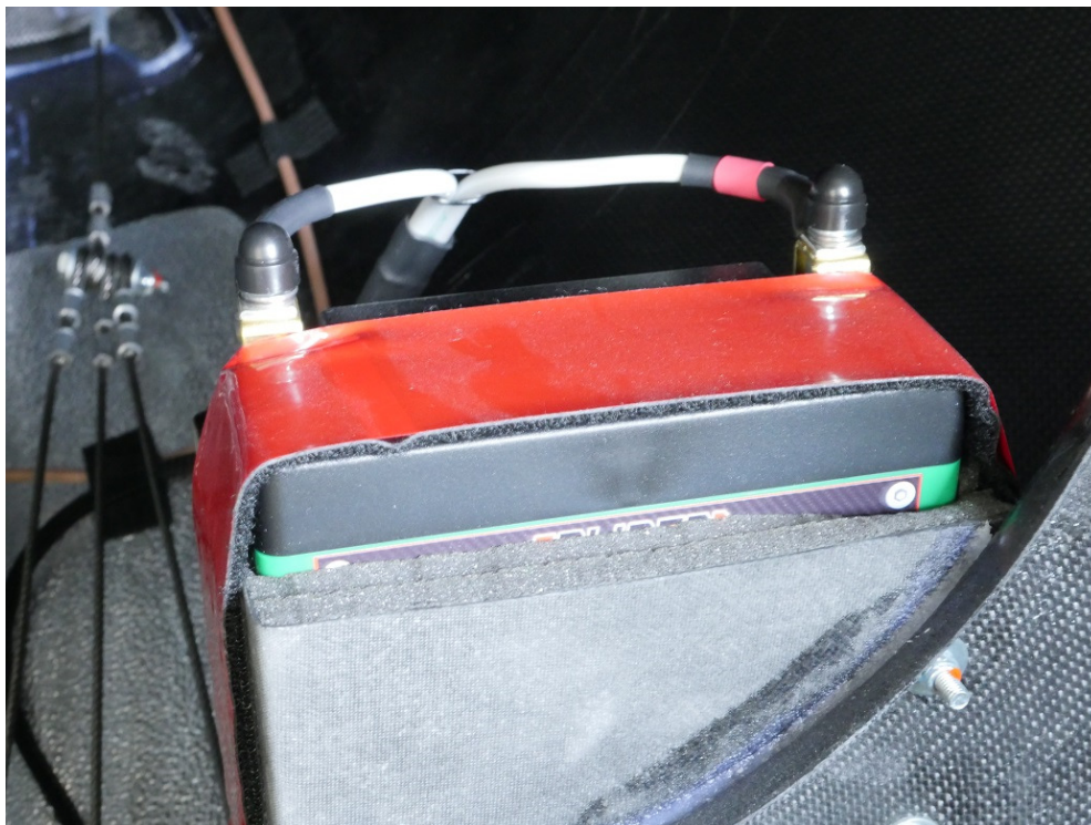
Figure 1: Aft battery installation
